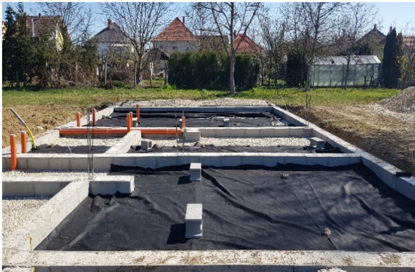
2: geotextile laying process
