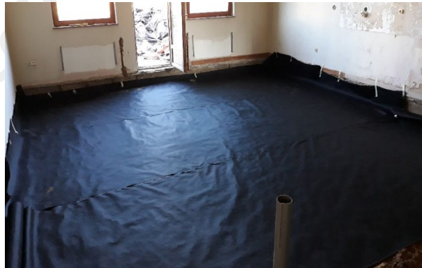
1: geotextile laying process
