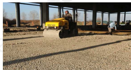
8: incorporation with a 3-tonne footpath roller
