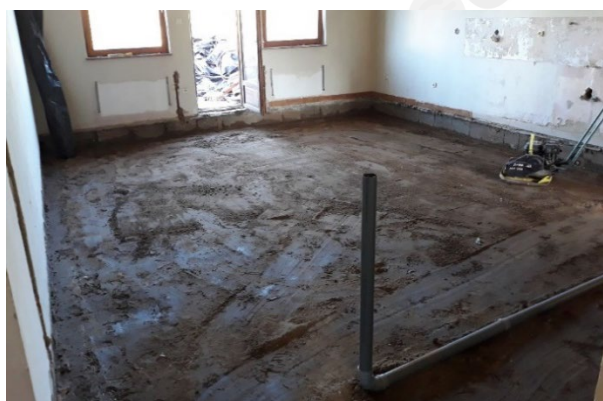
1: floor removed to the subsoil
