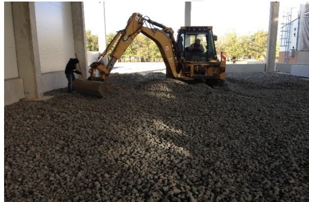
6: levelling out the foam glass layer with a front-end loader
