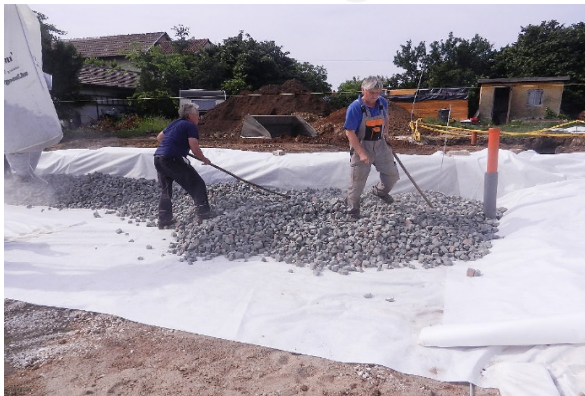
5: levelling out the foam glass layer with a rake
