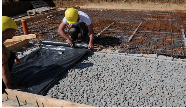
9: foam glass layer before placing the concrete
