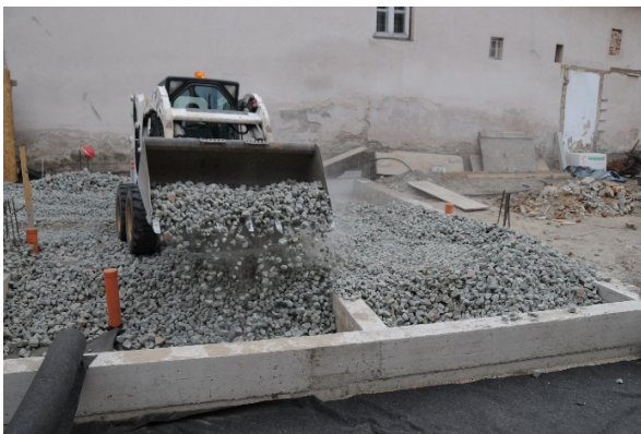
3: levelling out the foam glass layer with a small machine
