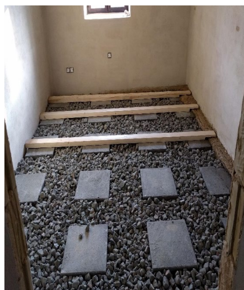
10: paving stones embedded in concrete, and vapour-permeable layer structure
