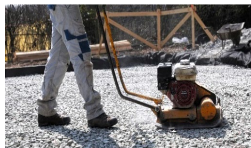
7: incorporation with a vibratory plate
